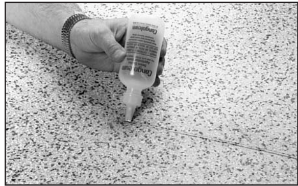
Fig. 8. Hold applicator bottle perpendicular to seam cut.
