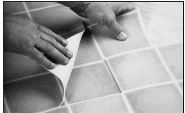
Fig. 112. Follow squared off edges to cut corner fill piece below.
