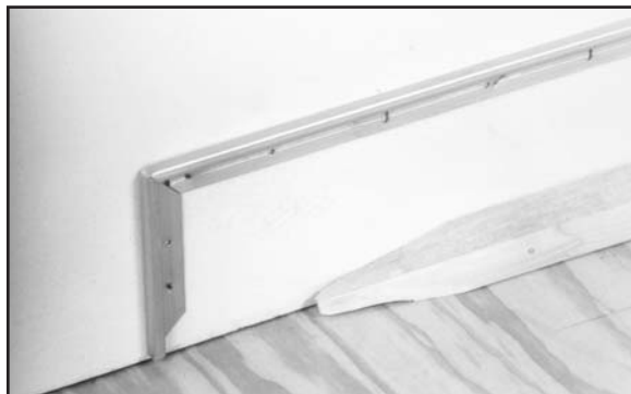
Fig. 99. Gradually taper cove fillet strip starting 2" to 3" (5.1cm to 7.6cm) from cap trim.
