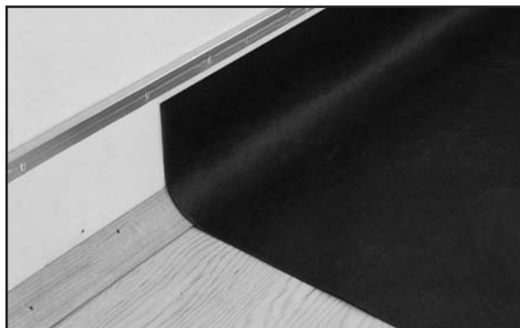
Fig. 101. Pattern felt must be held tightly against cove fillet strip and continue up wall to 1/4" (6.4mm) below cap trim.
