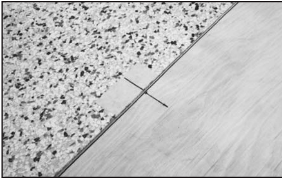
Fig. 113. Position flooring in room precisely on set marks.
