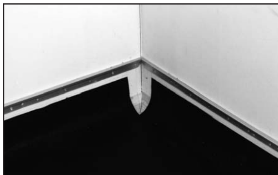
Fig. 102. Trim pattern felt about 1/2" (12.8mm) from inside corner juncture.
