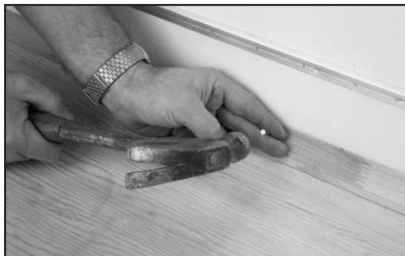
Fig. 100. Fasten cove fillet strip with nails (or other suitable fasteners) or adhesive.
