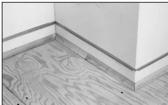
Fig. 98. Butt cove fillet strip tightly at inside and outside corners.
