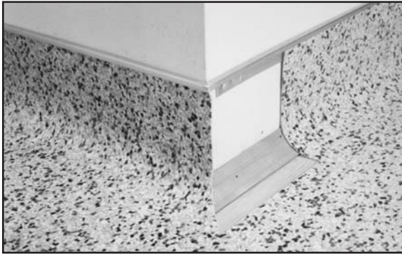
Fig. 114. Ready for completion of outside corner.
