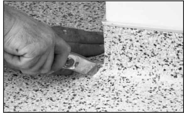
Fig. 116. Insert knife blade in cove fillet corner miter as a cutting guide.
